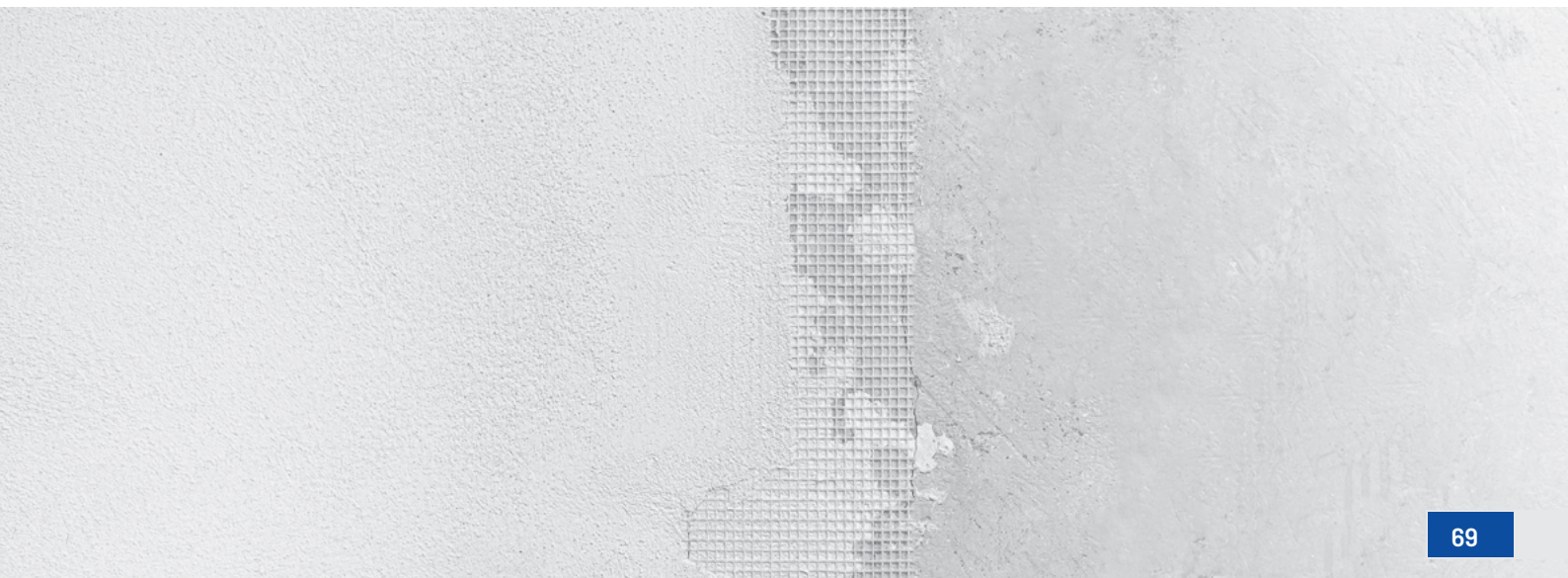
Reinforcing mesh used for strengthening of the waterproofing system
